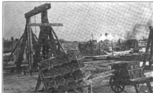
FIG. 2. LOADED PACKETS ON TWO-WHEEL BARROW; LOAD ABOUT 1,000 LBS.
